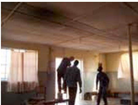
Kenny & Pastors Mathias & Chris working on the lighting system, Siphenzi.
